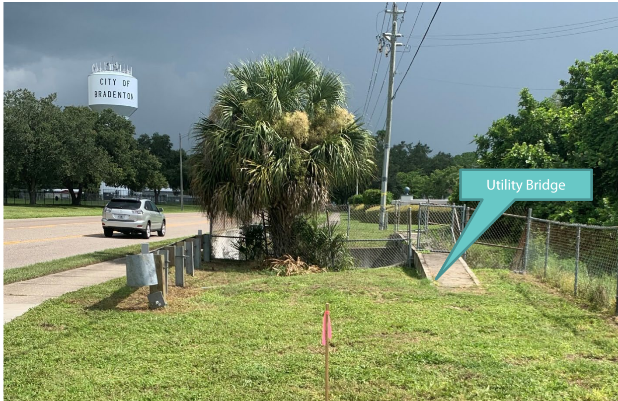
Figure 23: Utility Bridge over Cedar Hammock Creek (looking south)
