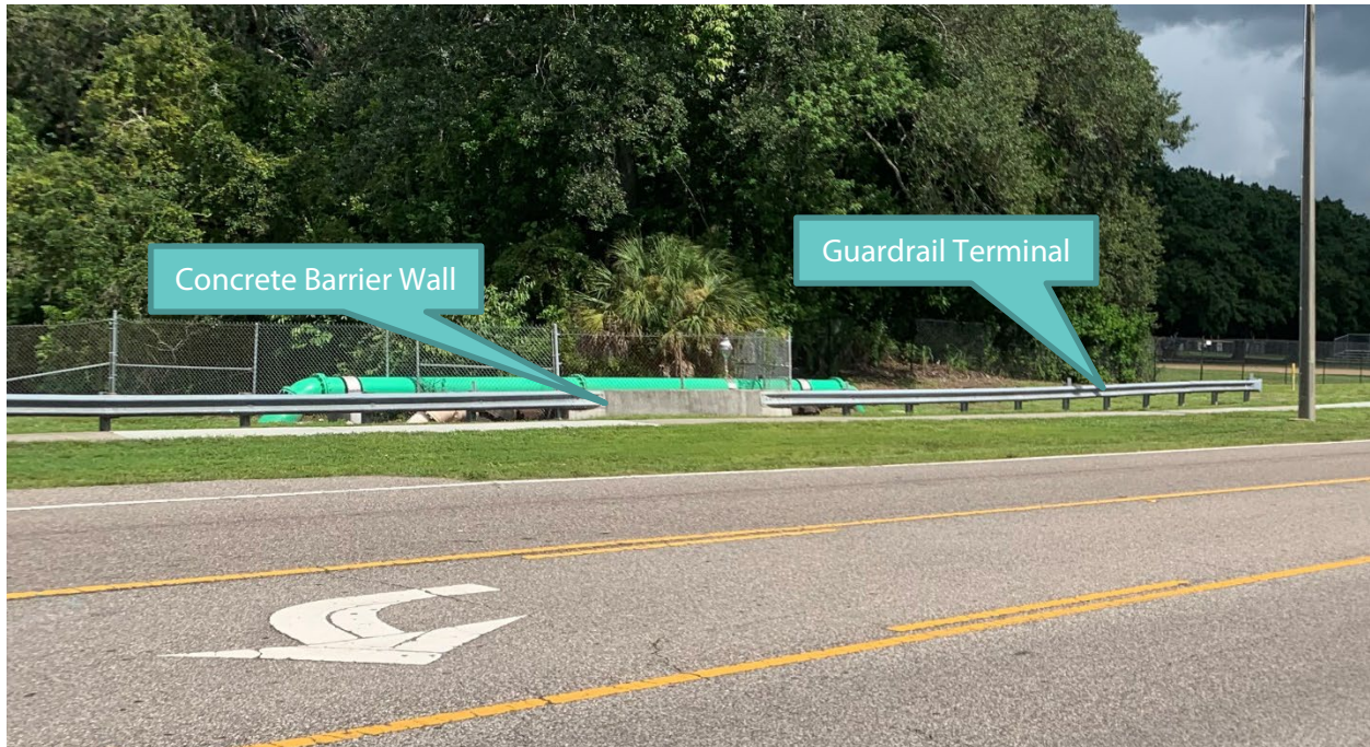
Figure 26: Culvert at Cedar Hammock Creek (looking east)
