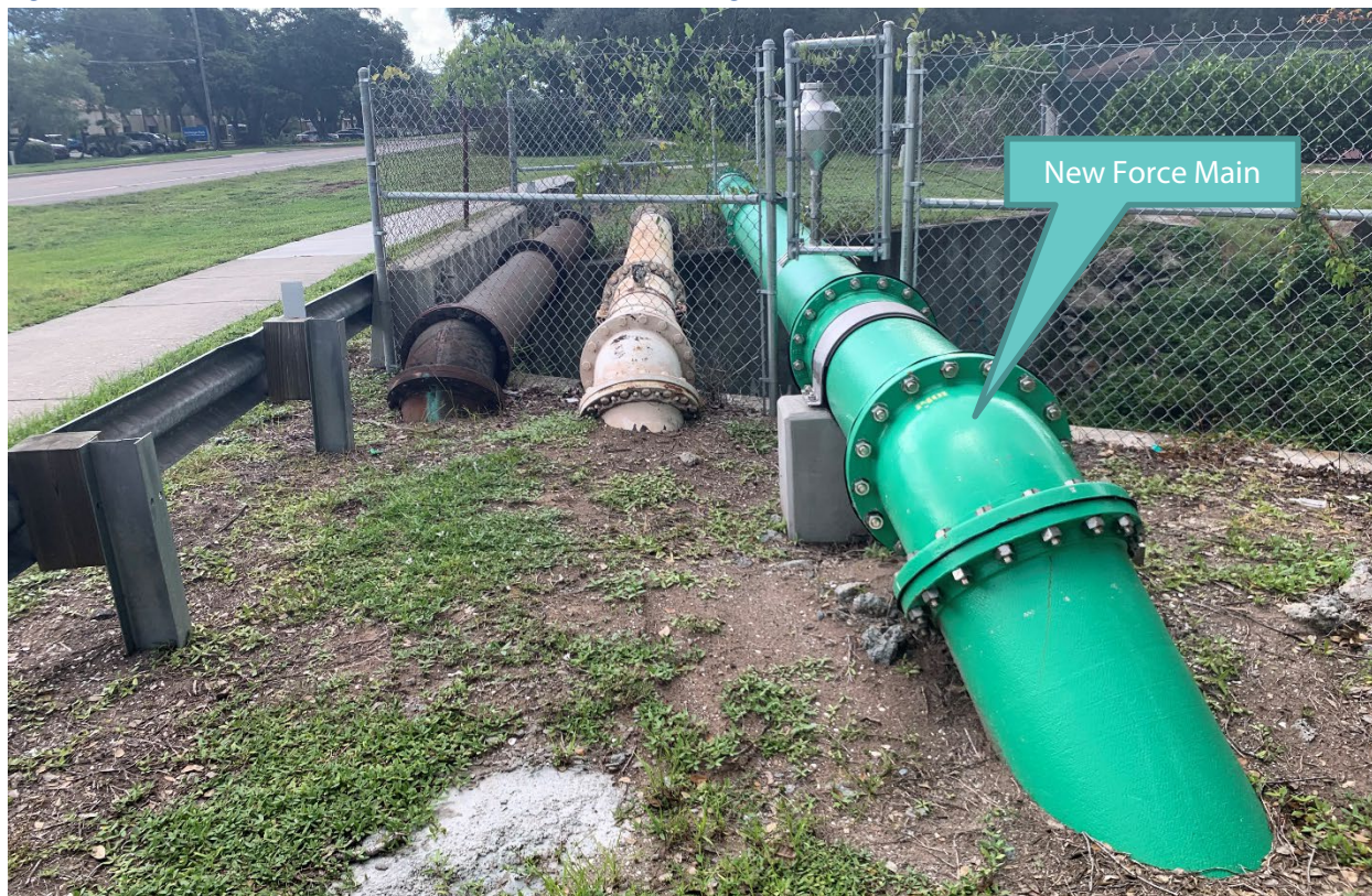
Figure 24: Utilities at Cedar Hammock Creek Culvert (looking north)
